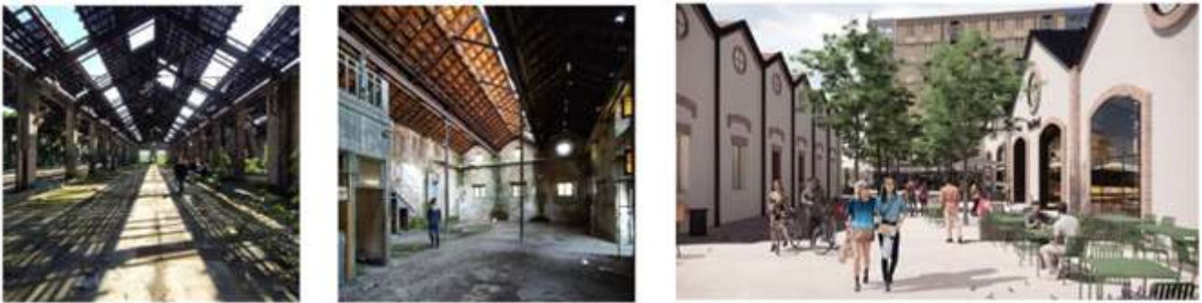
Figure 4: Scalo Porta Romana Milan. Two left pictures: before redevelopment. Right picture: after development (Scalo di Porta Romana, n.d.).
