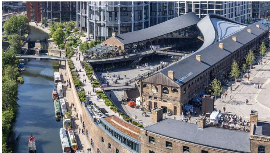
Figure 3: King's Cross Redevelopment London (Kings Cross, n.d.).
